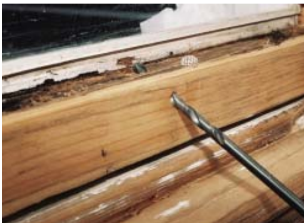
Figure 9. The bottoms of doors and windows are natural collection spots for moisture, but tiny vents allow the water to drain. Held in place by friction, the vents come in \frac{3}{8} -inch and \frac{1}{4} -inch sizes.
