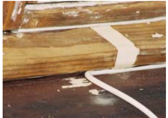
Figure 10. Designed for retrofitting weather stripping, this specialty tool cuts slots that are the perfect size for a caulked joint (left). The same manufacturer also makes the weather stripping that the author uses as a backer rod (above).
