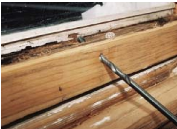
Figure 9. The bottoms of doors and windows are natural collection spots for moisture, but tiny vents allow the water to drain. Held in place by friction, the vents come in 3/8-inch and 1/4-inch sizes.
