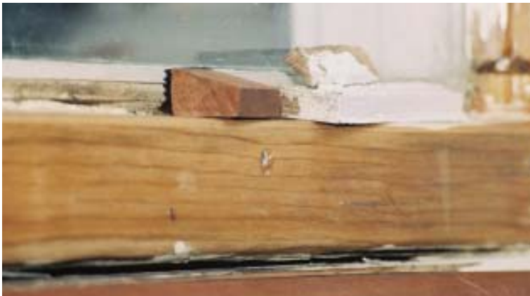
Figure 12. When the bottom stops on true-divided-light windows start showing the first signs of water damage, the author replaces them with wider versions cut from rot-resistant mahogany. Made with a steeper slope to aid in drainage, new stops are coated on all surfaces with two coats of epoxy. The black material on the front of the stop is a self-stick EPDM glazing gasket that the author uses instead of glazing putty.
