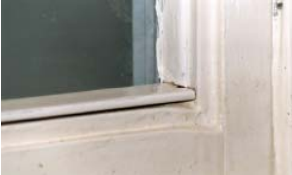
Figure 11. Mitered stops hold water, so the author copes new stops at the corners for better drainage, cutting the vertical stops — which are usually left in place — with a utility knife. Once installed, the new stops are sealed to the glass with silicone, the front edge is caulked with polyurethane, brad holes are filled with epoxy, and then the entire assembly is given another coat of Corlar 26P.
