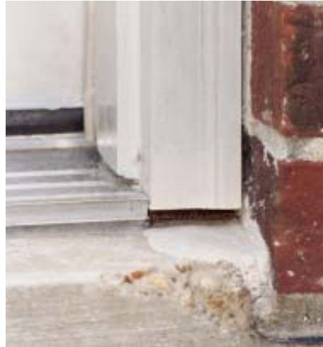
Figure 6. Before installing a door unit, the author likes to remove the brick molding, cut \frac{1}{8} inch to \frac{1}{4} inch off the bottom ends, coat them with epoxy, and staple bronze screening to them. Holes drilled in the trim at an upward angle and covered with small thimble vents allow interior moisture to drain while keeping out bugs.
