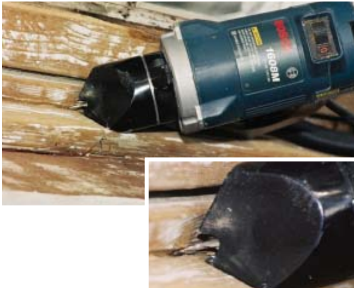
Figure 10. Designed for retrofitting weather stripping, this specialty tool cuts slots that are the perfect size for a caulked joint (left). The same manufacturer also makes the weather stripping that the author uses as a backer rod (above).
