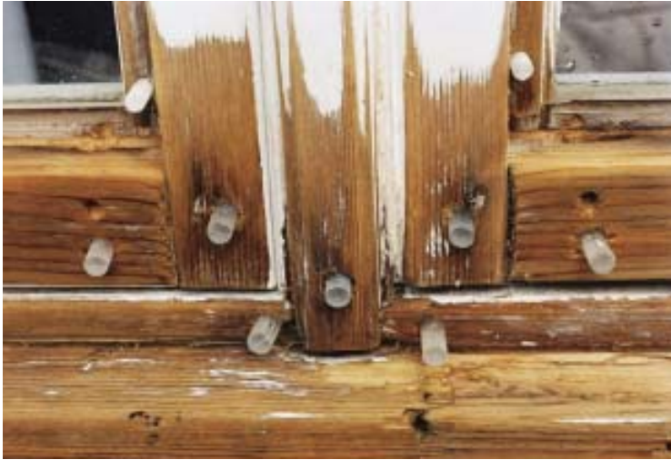
Figure 8. Made from compressed borax and available in different sizes, Impel Rods (above, right) can prevent rot. Inserted into vulnerable areas in windows and doors, the dowel-shaped pellets slowly dissolve when they're exposed to moisture, protecting the wood (above). The author uses a two-part epoxy wood filler — the same material used for repairs — to cap the holes.
