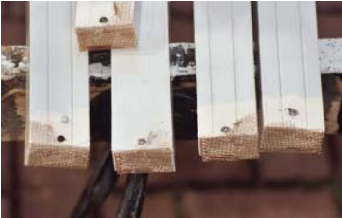
Figure 6. Before installing a door unit, the author likes to remove the brick molding, cut \frac{1}{8} inch to \frac{1}{4} inch off the bottom ends, coat them with epoxy, and staple bronze screening to them. Holes drilled in the trim at an upward angle and covered with small thimble vents allow interior moisture to drain while keeping out bugs.
