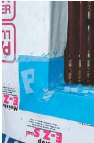
Figure 8. Sealing window flanges to the housewrap (far left) is a common practice, but it does not protect against the predictable leakage within the window assembly itself. Only a pan flashing that dumps on top of the drainage plane will effectively keep water out of the wall. Peel-and-stick membrane applied over the top of the building paper and wrapping the sides and bottom of the rough opening (left) accomplishes the task. Another option is Jamsill Guard, an injection-molded plastic sill pan with seamless corners, shown below. The author highly recommends Tyvek FlexWrap for pan flashings, whether the drainage plane is housewrap or rigid foam (below left).
