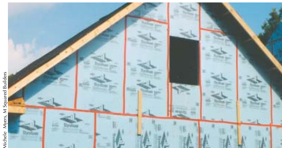
Figure 7. Extruded polystyrene or foil-faced polyethylene can be an effective drainage plane material. Joints in the foam can be taped with red Tyvek tape (top). To reduce reliance on tape or sealant, the author likes to apply the foam with shiplap joints at the vertical seams and a black poly strip as a Z-flashing at horizontal joints (right).
