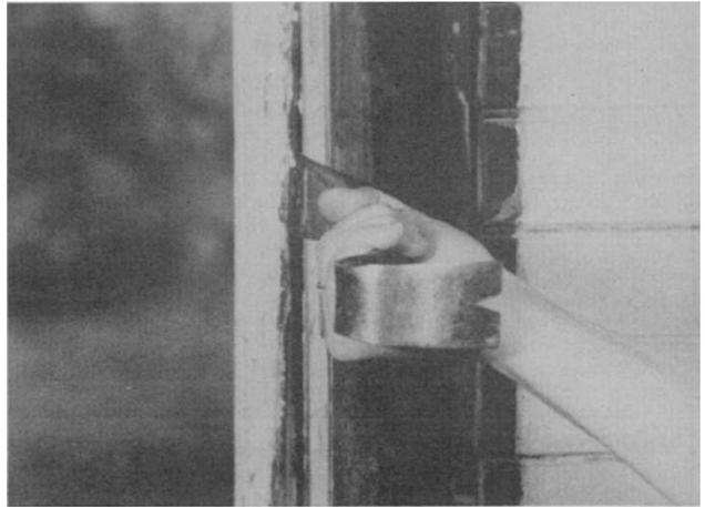
With a flat bar, pry off the parting bead to free the top sash.
