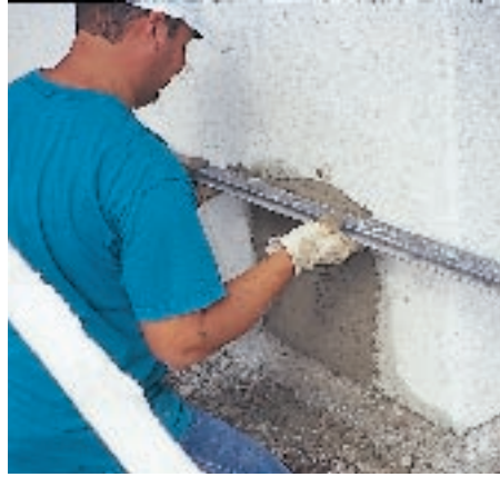
Figure 4. When patching, wet the surrounding stucco and apply an acrylic bonding agent. To keep the patch from sagging and shrinking, work the new stucco against the edges of the hole and apply the stucco in layers no more than 1/2-inch thick (left). Screenshot the final layer even with the surrounding stucco (middle), and touch up with the edge of a hand trowel (right).
