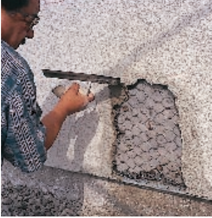
Figure 4. When patching, wet the surrounding stucco and apply an acrylic bonding agent. To keep the patch from sagging and shrinking, work the new stucco against the edges of the hole and apply the stucco in layers no more than 1/2-inch thick (left). Screenshot the final layer even with the surrounding stucco (middle), and touch up with the edge of a hand trowel (right).
