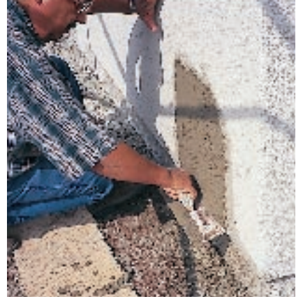
Figure 4. When patching, wet the surrounding stucco and apply an acrylic bonding agent. To keep the patch from sagging and shrinking, work the new stucco against the edges of the hole and apply the stucco in layers no more than 1/2-inch thick (left). Screenshot the final layer even with the surrounding stucco (middle), and touch up with the edge of a hand trowel (right).
