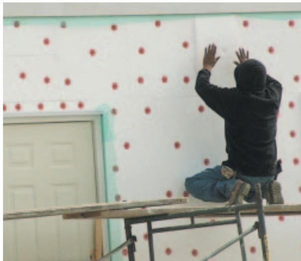
**Figure 2.** A worker attaches soft EPS "beadboard" with screws to form the base of the EIFS cladding. The close-up, below, shows the voids between the plastic beads. EPS allows water to leak through and can hold moisture against the building. That is why careful joint sealing and an effective secondary weather barrier are critical to system performance.
