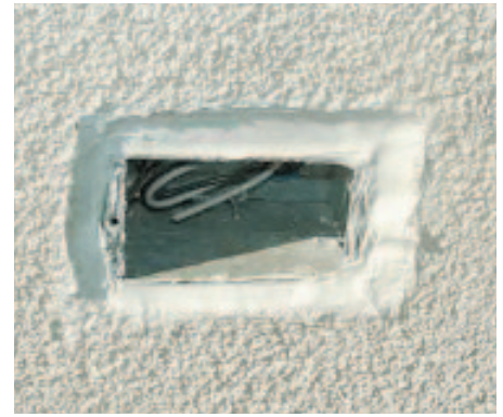
Figure 8. All penetrations should be flashed beneath the EIFS, as well as surface-sealed at the joint. In this example, peel-and-stick membrane is used to seal the electrical box to the housewrap (top left). A gap is left between the EIFS and the box (top middle), and the gap is then filled with backer rod and sealant (top right). Hose bibbs (left) receive a similar treatment.
