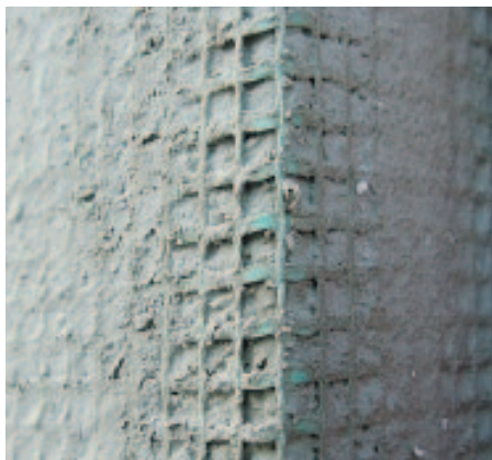
Figure 3. Woven reinforcing mesh (top left) serves to stop the cement and acrylic base coat from cracking. A coating protects the mesh against the alkaline cement, but mesh may still be weakened by moisture and chemical attack. A worker trowels the mesh into the wet base coat (above). For good coverage, the authors recommend applying the base coat in two layers: one layer before troweling in the mesh, and a second layer immediately afterward. Exposed mesh (bottom left) tends to lose strength over time.
