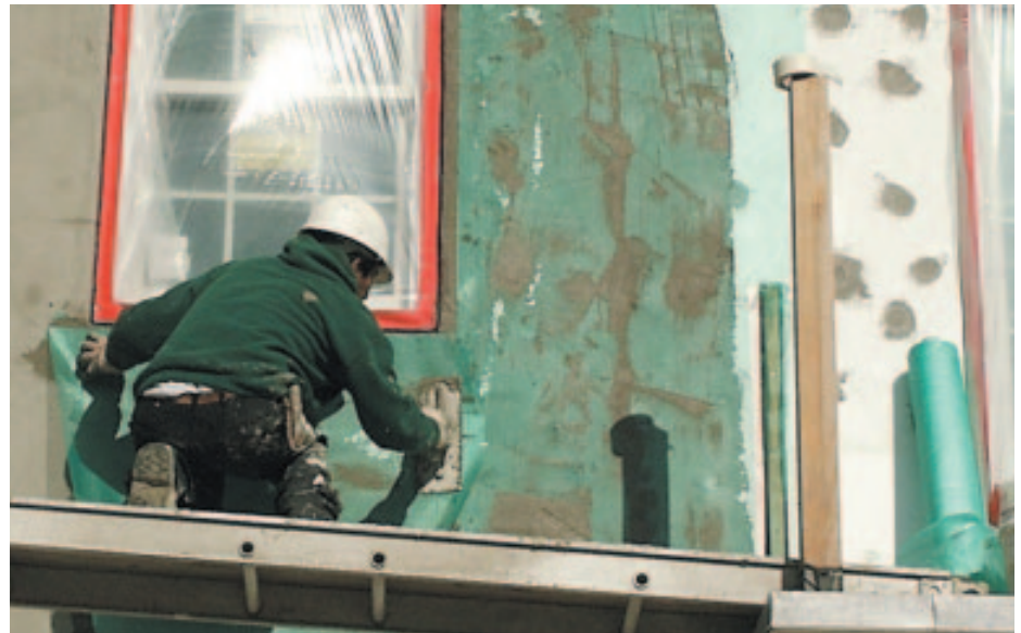
Figure 3. Woven reinforcing mesh (top left) serves to stop the cement and acrylic base coat from cracking. A coating protects the mesh against the alkaline cement, but mesh may still be weakened by moisture and chemical attack. A worker trowels the mesh into the wet base coat (above). For good coverage, the authors recommend applying the base coat in two layers: one layer before troweling in the mesh, and a second layer immediately afterward. Exposed mesh (bottom left) tends to lose strength over time.
