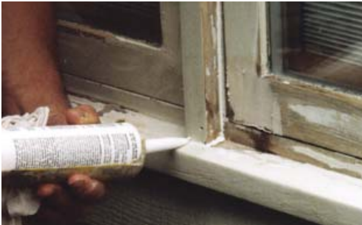
Figure 6. Careful caulking helps protect exterior joints and seams from water intrusion and future paint failure (above). Because horizontal surfaces are especially vulnerable, the author creates a fillet with caulk to help shed water: First, he applies a generous bead of caulk (above right), and then he smooths out the surface with his dampened finger (right).
