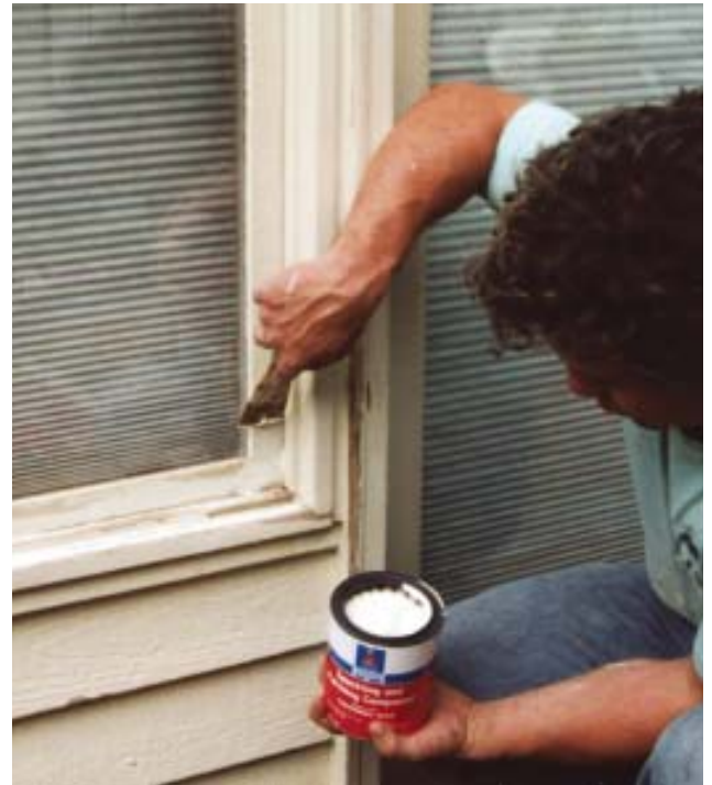
Figure 3. After scraping, the author fills small holes and minor gouges with a quick-drying spackling compound.
