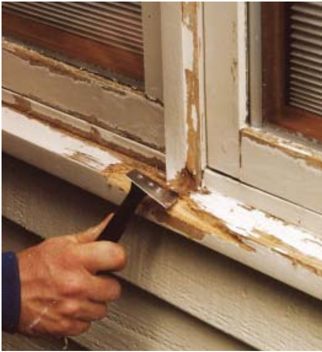
Figure 2. Scraping wood windows before they are repainted removes disbonded paint and reveals areas where rot has taken hold.
