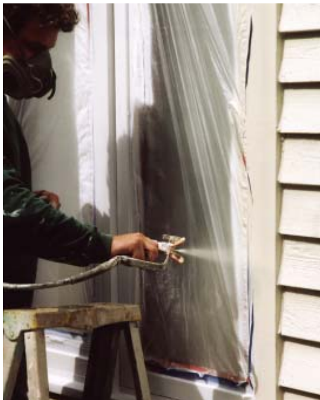
Figure 11. After spraying on the window's finish coat (above) — and allowing enough drying time, so that the tape won't lift the paint — the author masks around the frame with regular tape, tucking plastic underneath (above right), before finishing the rest of the siding (right).
