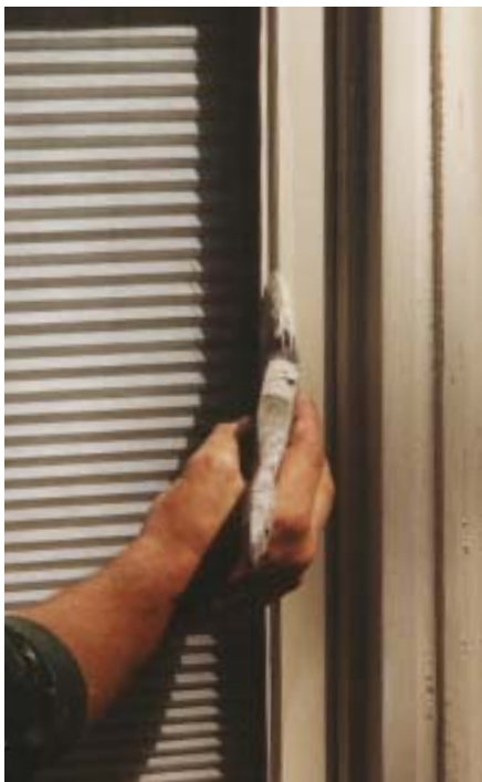
Figure 8. Using a 3 1 / 2 -inch angled sash brush, the author laps the paint slightly onto the glass, creating a final barrier against water intrusion.
