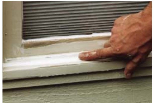
Figure 6. Careful caulking helps protect exterior joints and seams from water intrusion and future paint failure (above). Because horizontal surfaces are especially vulnerable, the author creates a fillet with caulk to help shed water: First, he applies a generous bead of caulk (above right), and then he smooths out the surface with his dampened finger (right).
