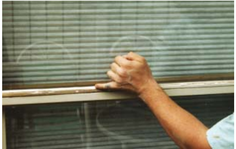
Figure 7. To prevent water from running behind the glazing trim, the author caulks this joint around all four sides of each window, paying particular attention to the bottom rail, where water intrusion is most likely (left). A slightly dampened little finger is useful for tooling this joint smooth (above).
