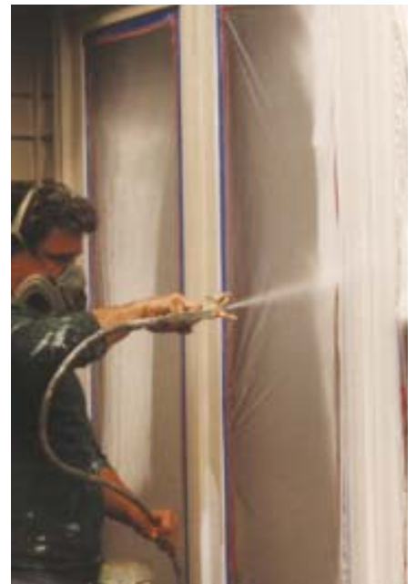
Figure 10. To minimize sag-producing crossing patterns, the author makes quick vertical passes with his spray gun and sprays lightly, sometimes applying two thinner coats rather than a heavier one that may need to be brushed out.
