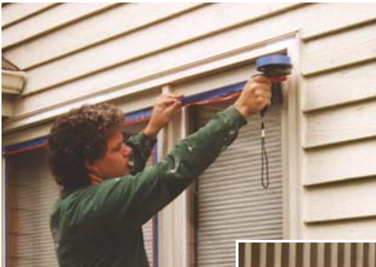
Figure 9. Spraying is considerably faster than brushing when windows, siding, and trim are being painted at the same time. The author begins by using a dual-tack tape dispenser to mask the window glass (above), being careful to leave a slight, even gap between the tape and glazing trim (inset). Then he lays painter's plastic onto the tape, trimming it to size with a razor blade (far right).
