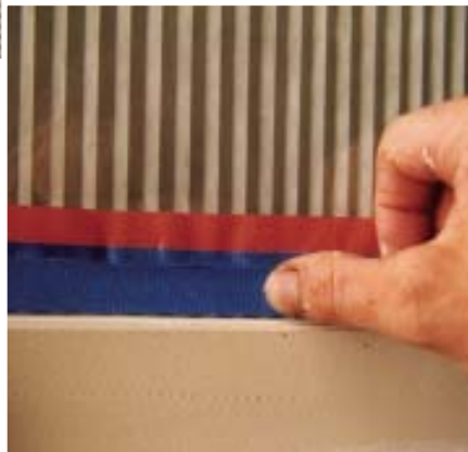
Figure 9. Spraying is considerably faster than brushing when windows, siding, and trim are being painted at the same time. The author begins by using a dual-tack tape dispenser to mask the window glass (above), being careful to leave a slight, even gap between the tape and glazing trim (inset). Then he lays painter's plastic onto the tape, trimming it to size with a razor blade (far right).
