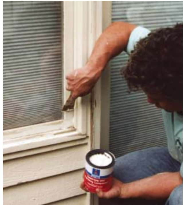
Figure 3. After scraping, the author fills small holes and minor gouges with a quick-drying spackling compound.
