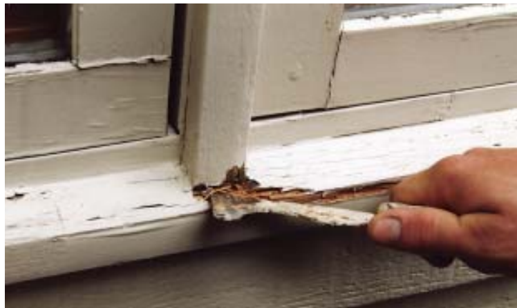
Figure 1. Some wood windows are built with sills that have no slope — or even a reverse slope — which means water can't easily drain away from the glazing (left). Instead, it gets absorbed by the end grain of vertical window components that sit on the sill, quickly leading to paint failure and rot (above).
