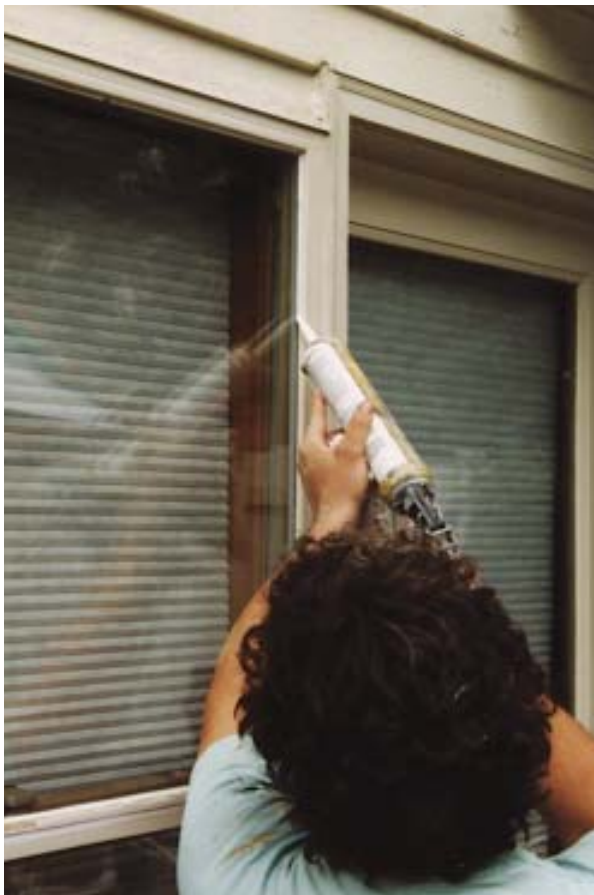
Figure 7. To prevent water from running behind the glazing trim, the author caulks this joint around all four sides of each window, paying particular attention to the bottom rail, where water intrusion is most likely (left). A slightly dampened little finger is useful for tooling this joint smooth (above).
