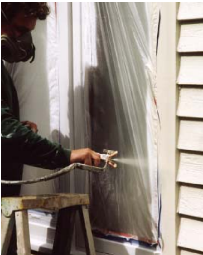
Figure 11. After spraying on the window's finish coat (above) — and allowing enough drying time, so that the tape won't lift the paint — the author masks around the frame with regular tape, tucking plastic underneath (above right), before finishing the rest of the siding (right).
