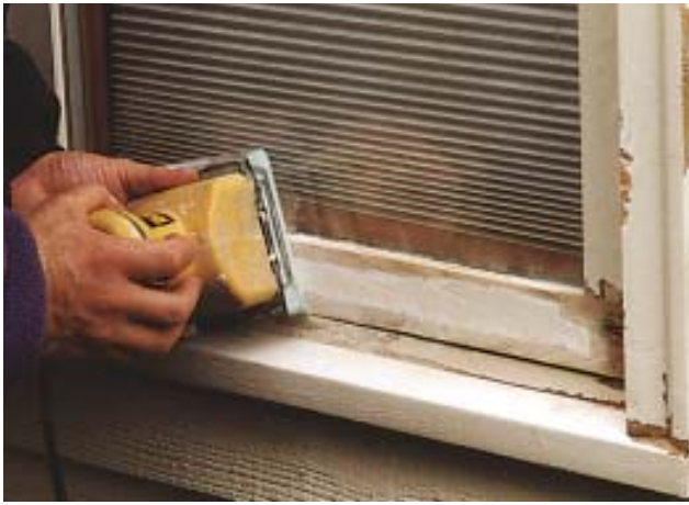
Figure 5. After the scraping and epoxy repair work, a palm sander loaded with 60-grit paper smooths the wood surface, feathering out the old paint and rounding over sharp edges. New unprimed windows should also be scuff-sanded to remove mill glaze.
