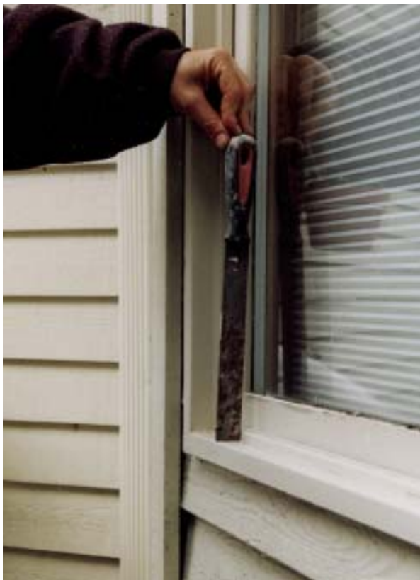
Figure 1. Some wood windows are built with sills that have no slope — or even a reverse slope — which means water can't easily drain away from the glazing (left). Instead, it gets absorbed by the end grain of vertical window components that sit on the sill, quickly leading to paint failure and rot (above).
