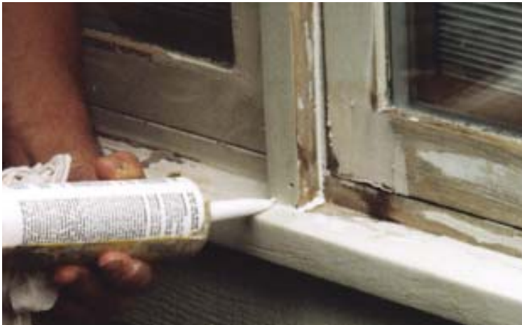
Figure 6. Careful caulking helps protect exterior joints and seams from water intrusion and future paint failure (above). Because horizontal surfaces are especially vulnerable, the author creates a fillet with caulk to help shed water: First, he applies a generous bead of caulk (above right), and then he smooths out the surface with his dampened finger (right).
