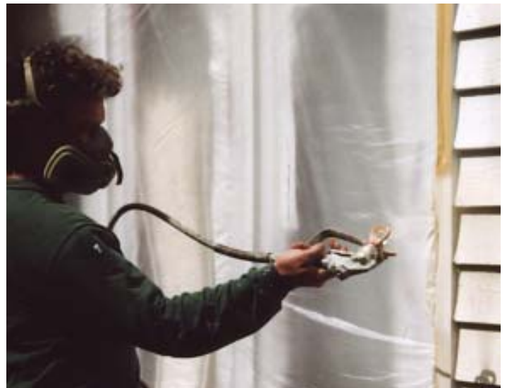
Figure 11. After spraying on the window's finish coat (above) — and allowing enough drying time, so that the tape won't lift the paint — the author masks around the frame with regular tape, tucking plastic underneath (above right), before finishing the rest of the siding (right).
