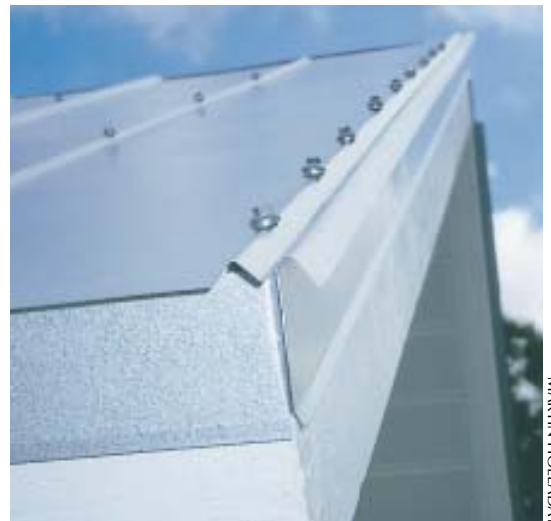
Figure 2. Many installers put screws in the ribs even though manufacturers discourage it. The practice is a holdover from when the dominant fasteners were nails. Using screws and installing them in the flat sections of the panel is considered a better practice by manufacturers, because of screws' lower shear strength and better sealing compared to nails.
