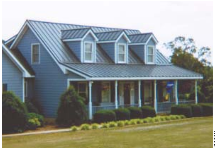
Figure 1. Exposed-fastener metal roofing has long been used for barns and industrial buildings because it's inexpensive, installs quickly, and lasts 30 or 40 years. It also makes a great residential roof in areas with a rural character, especially in hot or snowy regions.
