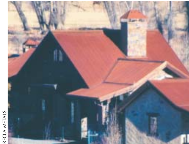
Figure 11. Using uncoated or Cor-Ten steel roofing helps new buildings fit in with historic surroundings. This exposed-fastener roof uses plain cold-rolled steel, but Cor-Ten steel, more traditionally used on bridges and guardrails, creates a similar look.
