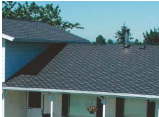
Figure 7. Modular roofing products, the fastest-growing segment of the metal roofing industry, fit well in older neighborhoods. They blend easily with more conventional roofing materials like asphalt, cedar shingles, and concrete tile but offer the longevity, durability, and weight advantage of metal. Clockwise from left are the Tasman Decra Shingle, ASC Tek Guard, and GP Centura.
