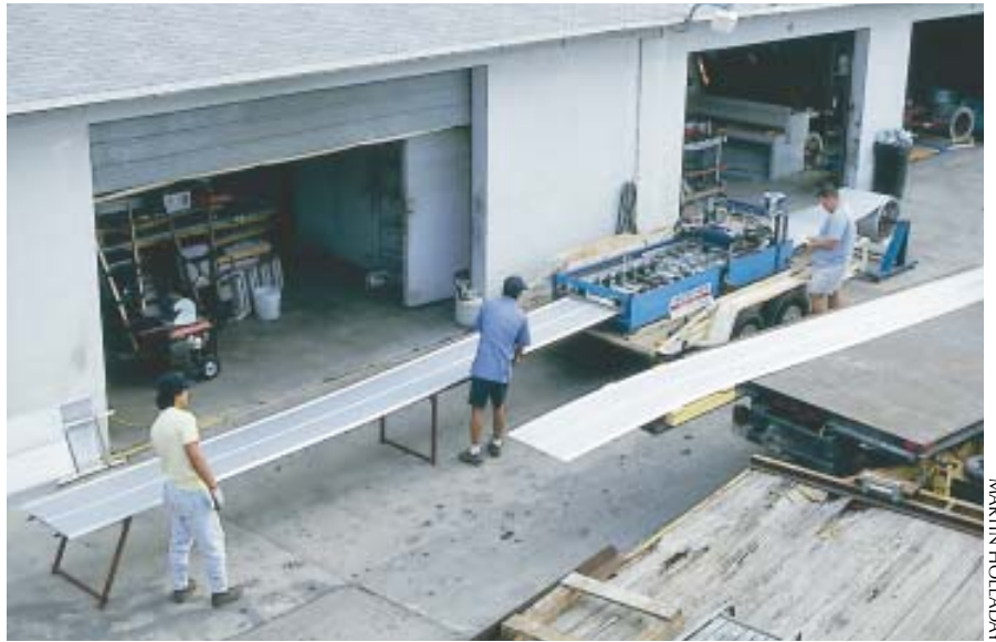
Figure 5. Forming standing-seam panels on site used to mean folding and crimping sheet stock with hand tools, but modern tow-behind roll-forming equipment can quickly make standing-seam and exposed-fastener panels to virtually any length.
