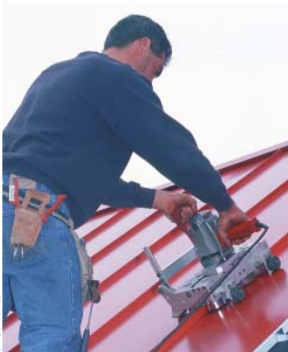
Figure 6. Motorized crimpers (left) seam panels with little effort but lots of time. Manufacturers are now producing snap-together panels that look hand-seamed but install faster (above).
