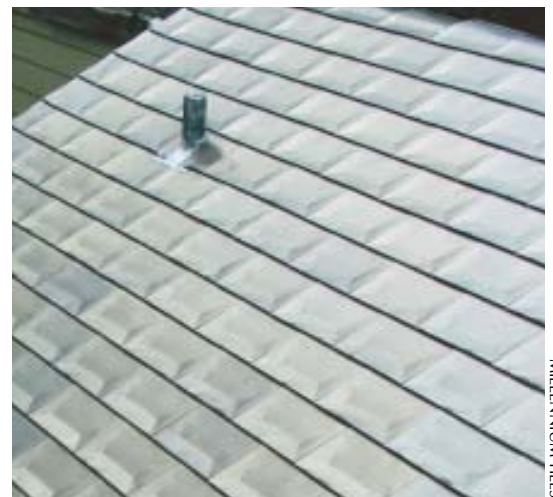
Figure 15. Offering the greatest corrosion protection possible, recently introduced stainless modular shingles look modern and seem ideal for coastal areas, where salt spray corrodes other metals.
