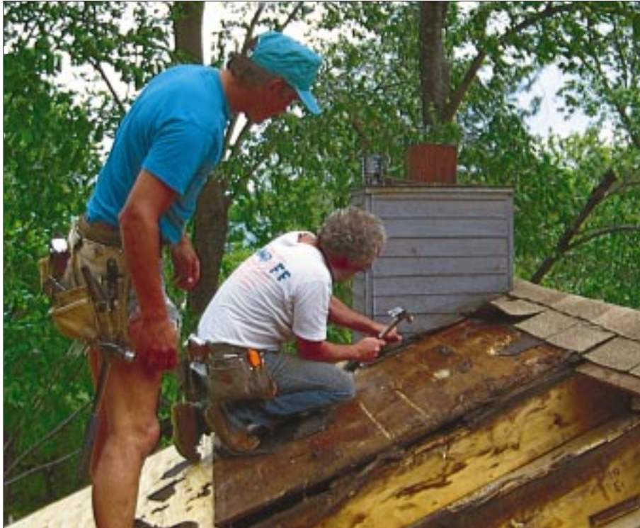
Workers tear off rotten sheathing over an unvented cathedral ceiling.
