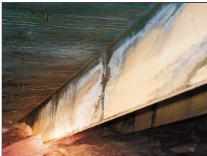
Figure 1. Moisture trapped in the attic raised the moisture content of the wood to well over 20%. Vigorous growth of several types of fungi turned the underside of the roof sheathing completely black.
